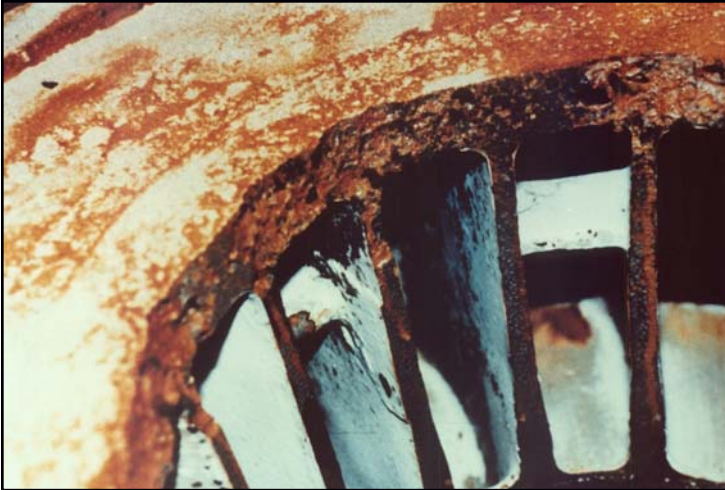
Corroded Rotor Taper
